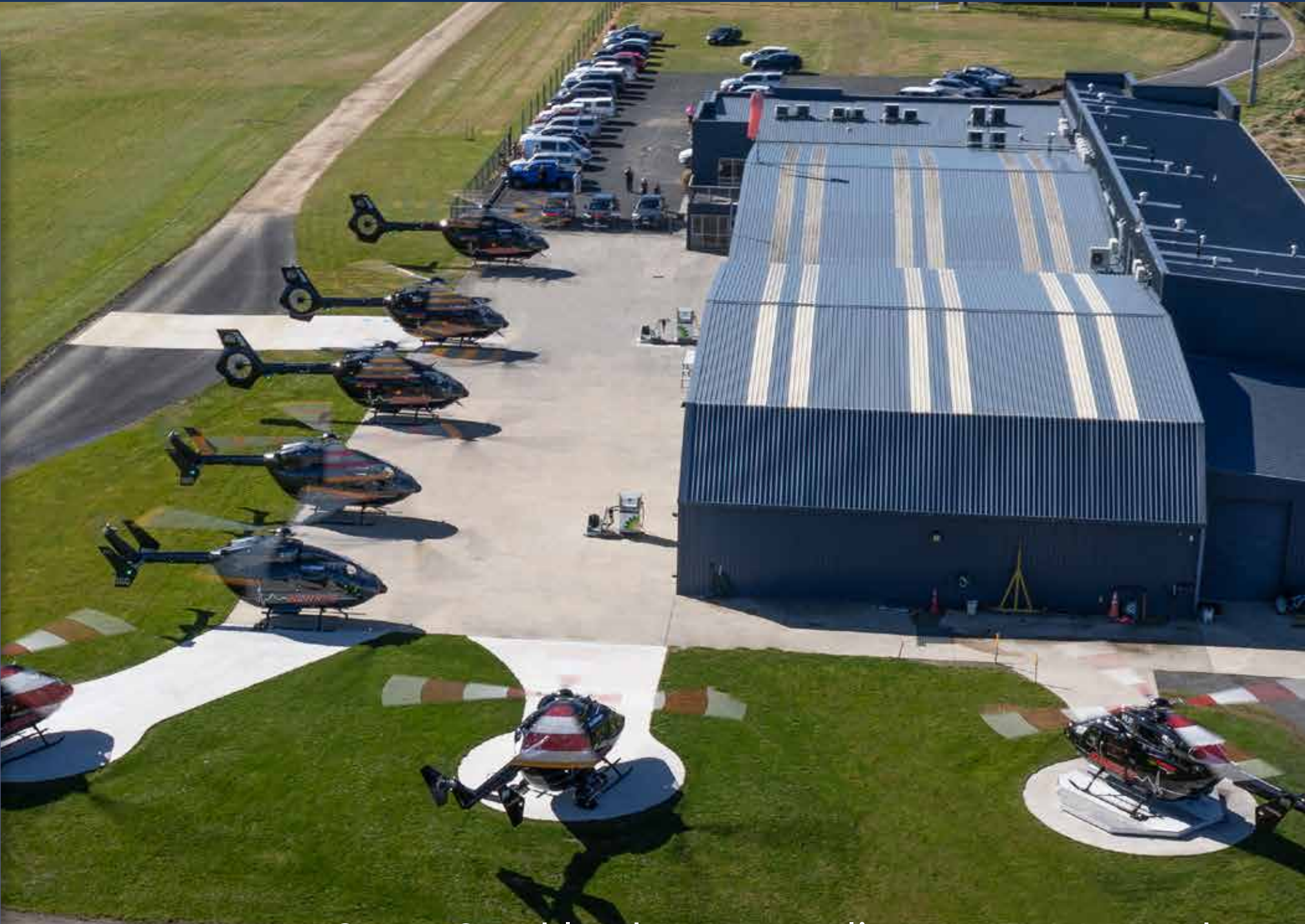
Otago Southland Rescue Helicopter Trust Board
